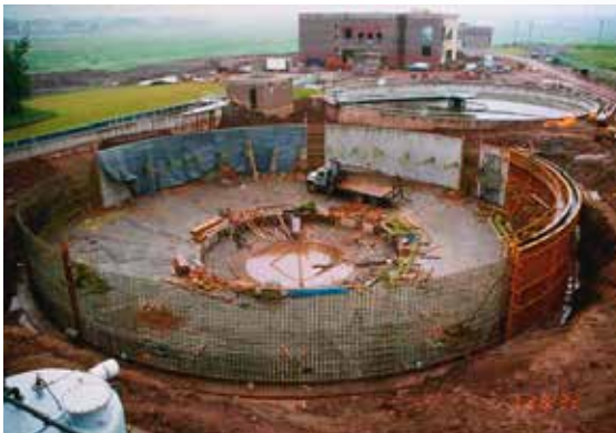
Clarifier under construction.
