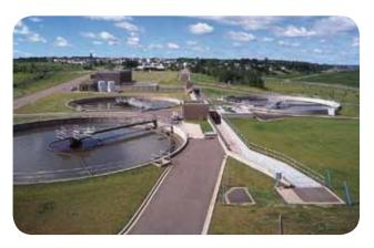
The actual WWTF was commissioned in 1994 with a capacity of 115,000 m³ per day, or 25 million gallons per day. The plant was laid out to facilitate expansion to biological treatment in the future.
