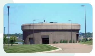
The Main Pumping Station located on the plant site at Outhouse Point (property having been granted initially to a Mr. Robert Outhouse) is the heart of the collector sewer system, a point of collection for all lines and continuous pumping to the Wastewater Treatment Facility (WWTF). The cylindrical structure extends 30 m below grade and 9 m above ground, much like a 10-storey building underground.
